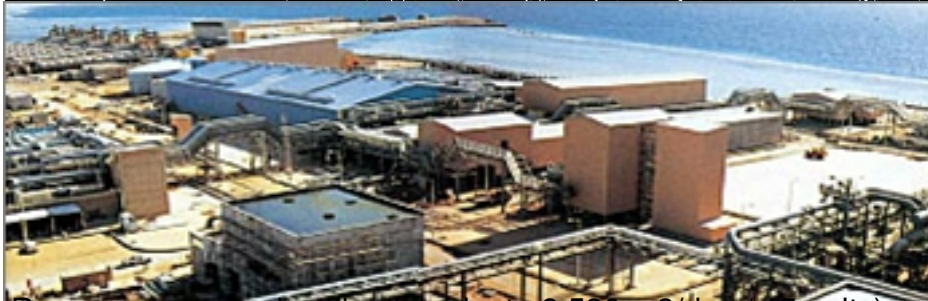
Reverse osmosis desalination plant (8 530 m 3 /day / 15 units)
