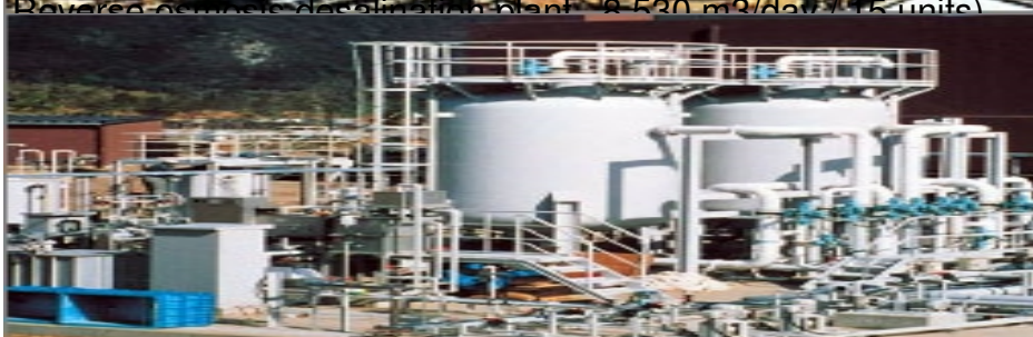
Reverse osmosis desalination plant (HUIS TEN BOSCH, 500 m 3 /day / 2 units)
